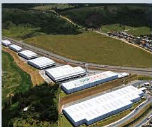
LOG VIA EXPRESSA - MG
